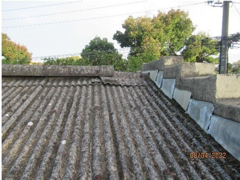
Corrugated roof sheeting
